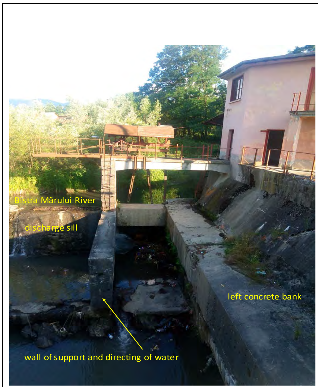
Figure 24: The discharge sill of the lower Bistra Mărului River sector.
